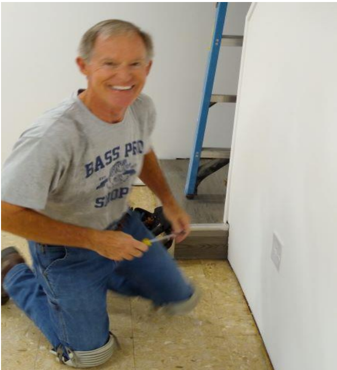
Doug Woody is installing electrical plates on outlets.
